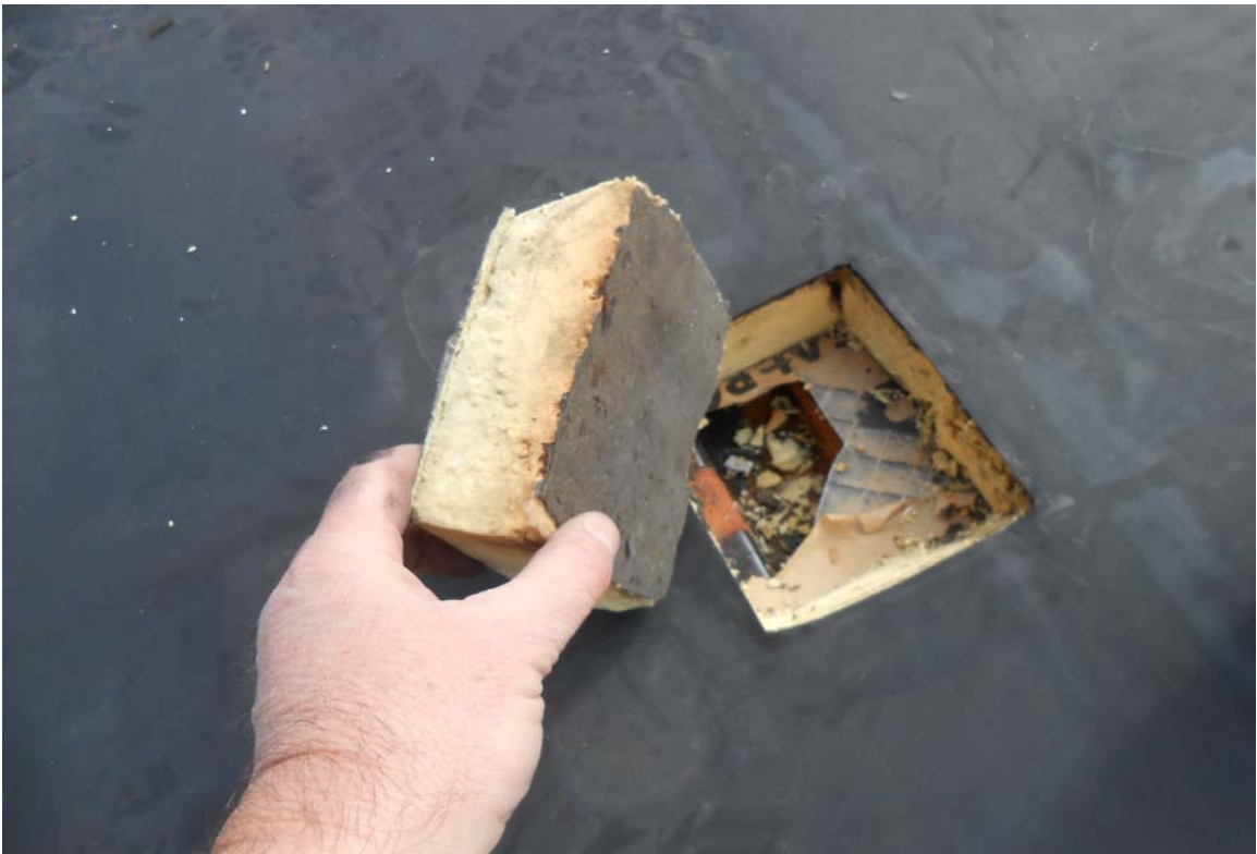
Picture No. 2 – Sample test cut of the upper roof level.
