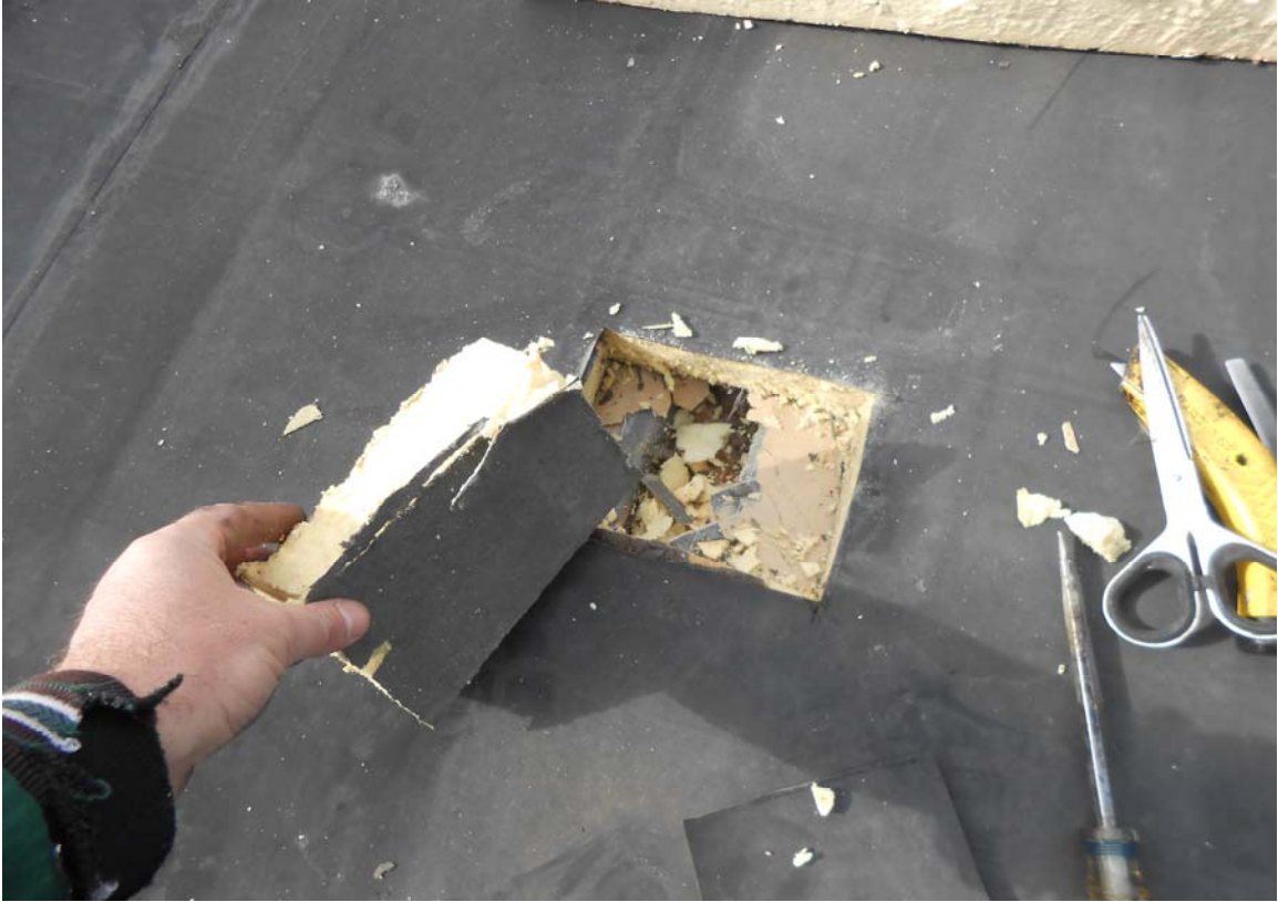
Picture No. 1 – Sample test cut of the lower roof level.
