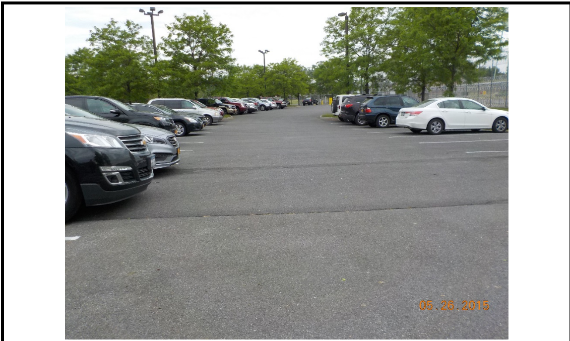
Photograph #4 - Description: Observed patch at southwestern parking lot, looking south.
