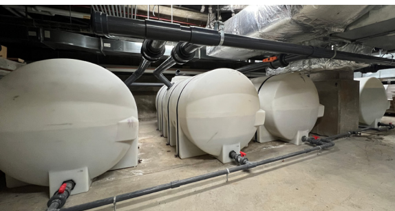
ESF's (SUNY) rainwater recovery system has reclaimed more than 4,300 gallons of water used to wash vehicles, water plants, and for other general purposes on campus over the past three years. Credit: SUNY ESF
