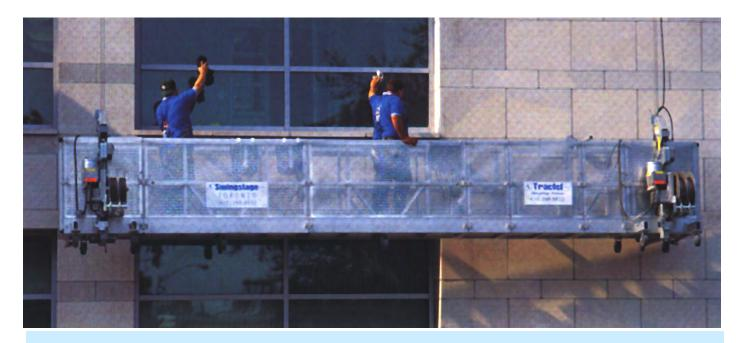
**Powered platforms** are the most popular solution for exterior building access in North America.
