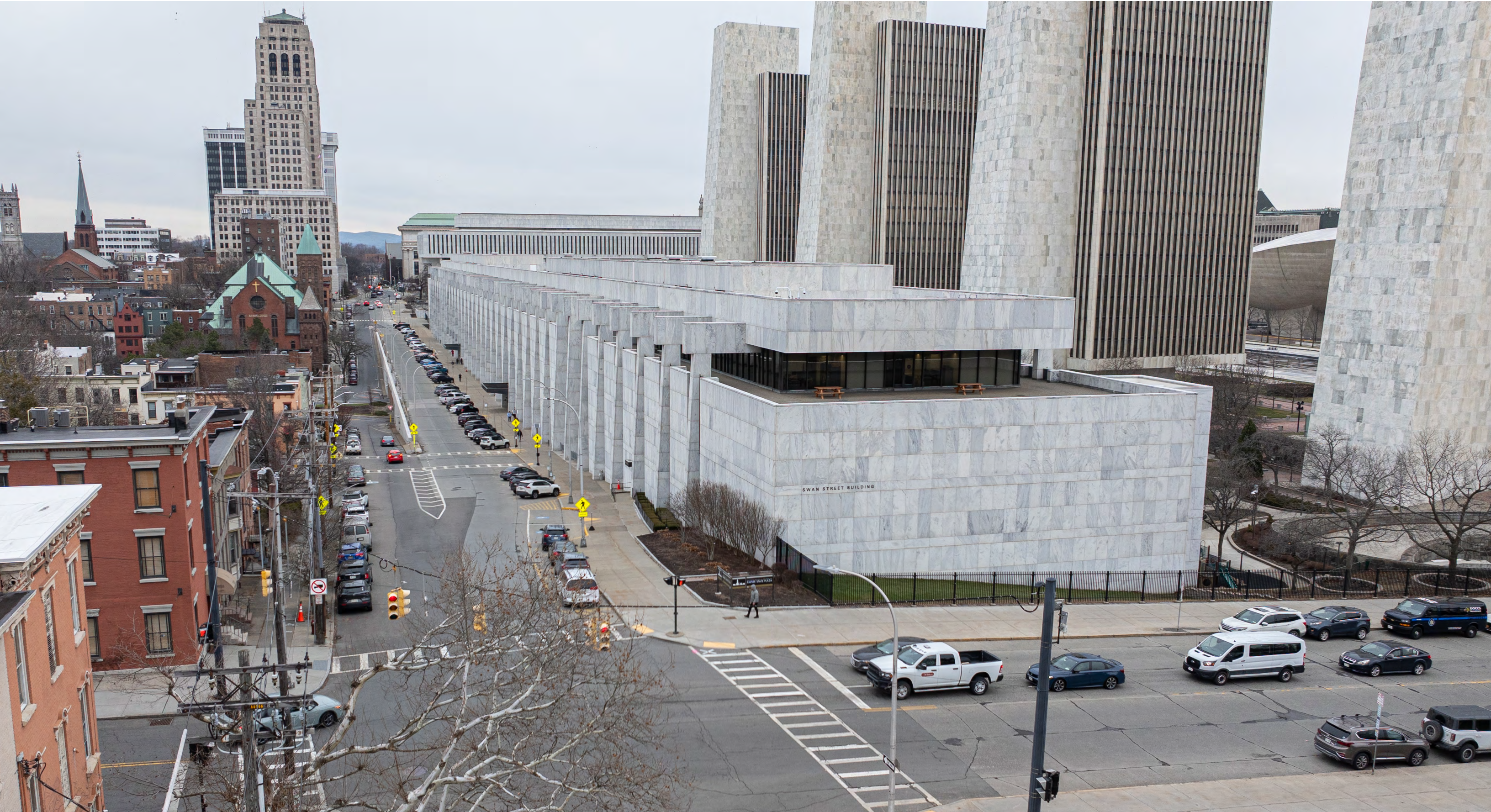
Swan Street, Existing Condition
