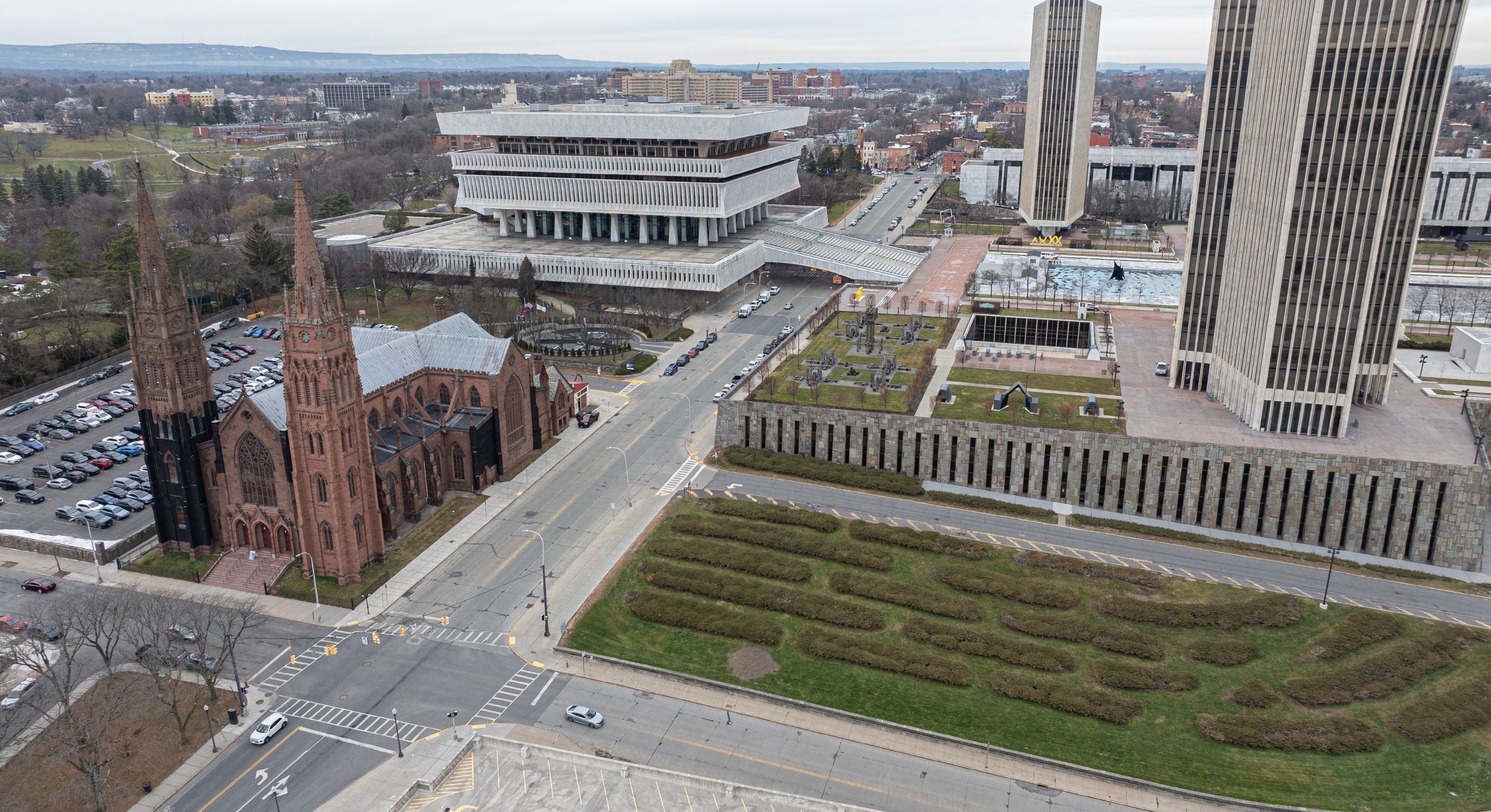
Madison Avenue, Existing Condition
