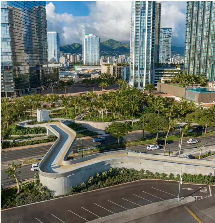
Ala Moana Boulevard Pedestrian Bridge Honolulu, HI
